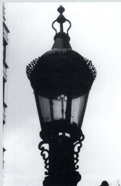
This handsome gas lamp in Carting Lane dates from 1900. Burning night and day, its purpose is to extract and burn methane originating from a nearby sewer.
